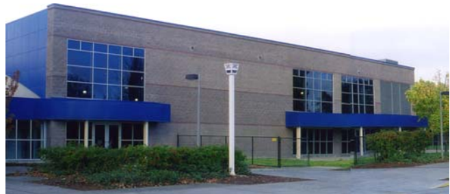
Fig. 1: East Wall of Aquatic Center
