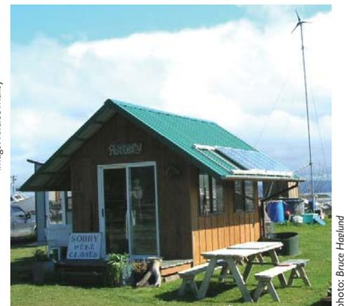
This self-sufficient potter's studio in Nachotta, WA, epitomizes the concept of site-generated energy—PVs and a wind turbine to run the lights and kiln, as well as effective shading.
