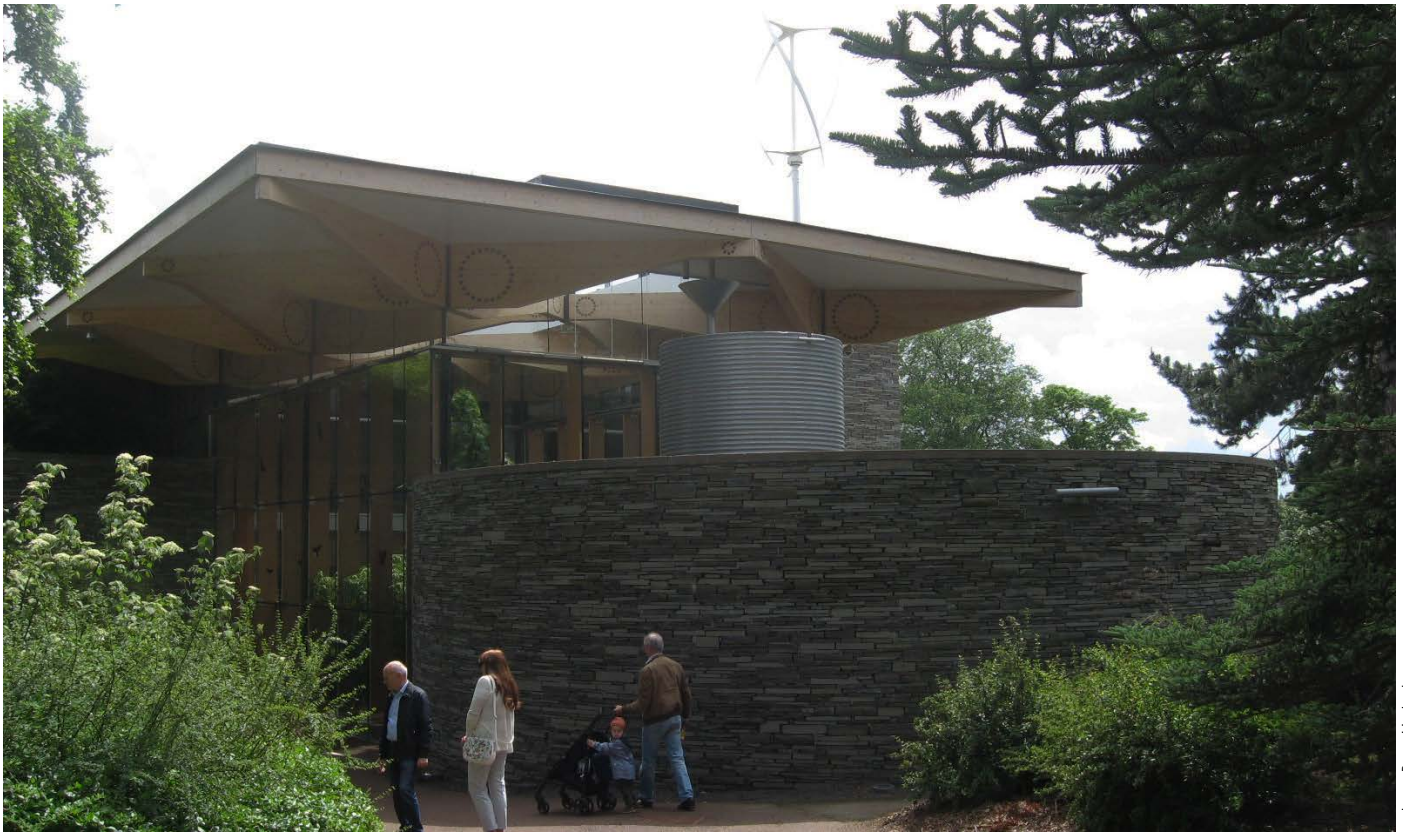
A backside view of the Hope Gateway reveals the wind turbine, glulams, the atrium entry, and the cistern perched above the loos clad in local stone.
